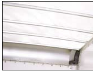
Translucent roof brightens interior.
